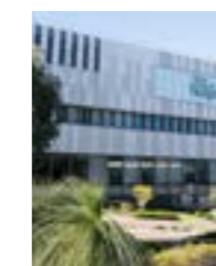
Fiona Stanley Hospital
